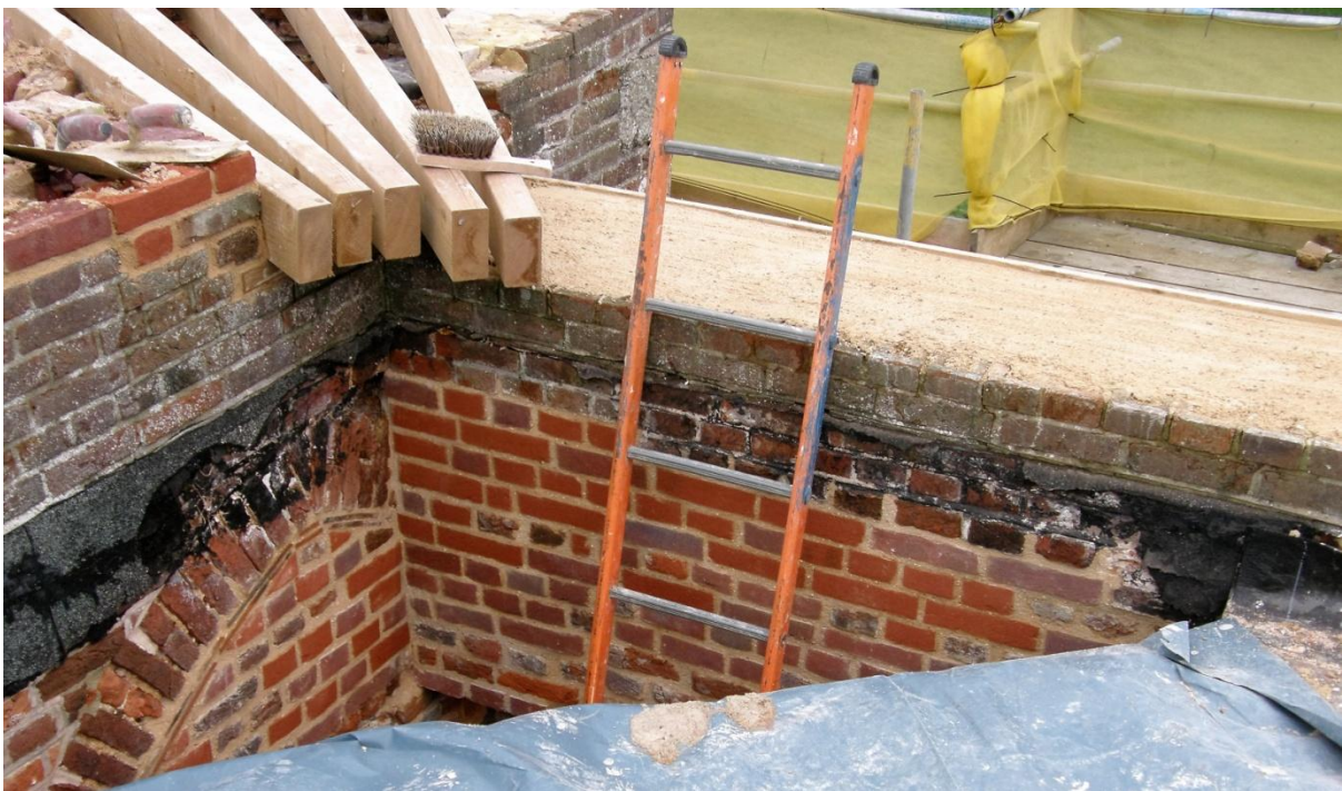
4: - and today, with it re-built with new bricks and lime mortar
