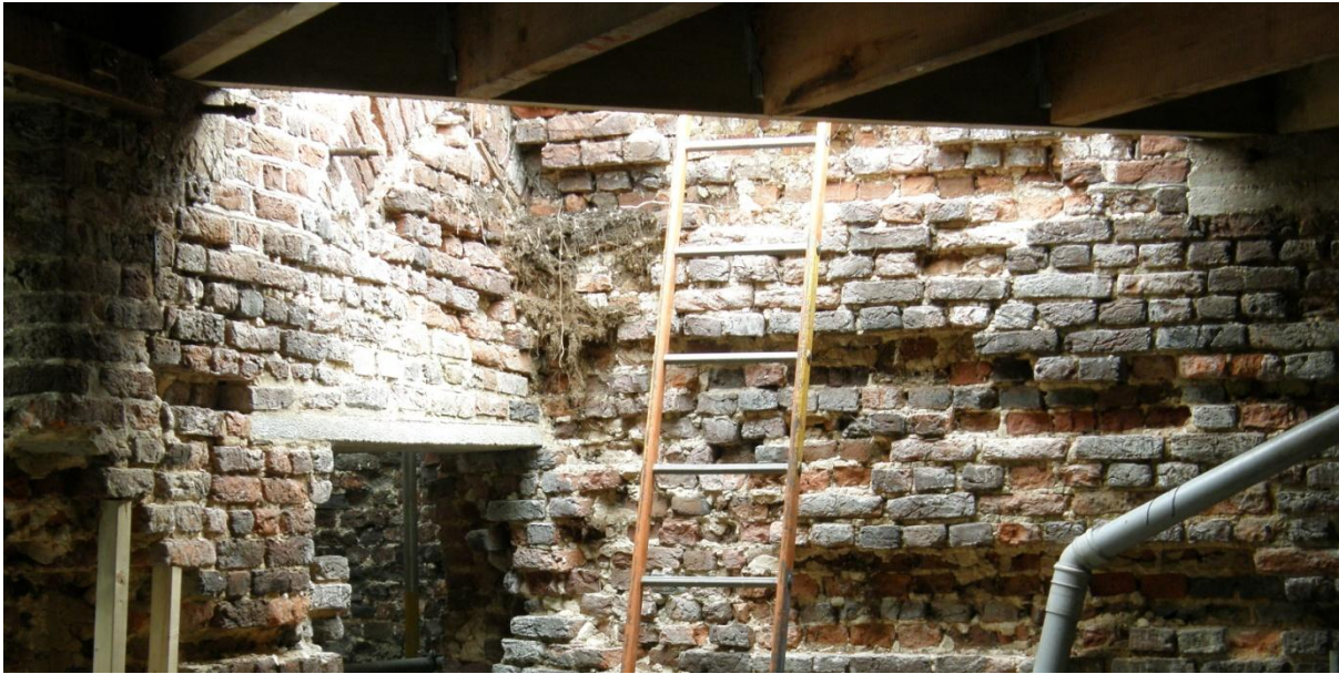
3: The upper brickwork below the roof in a state of collapse
