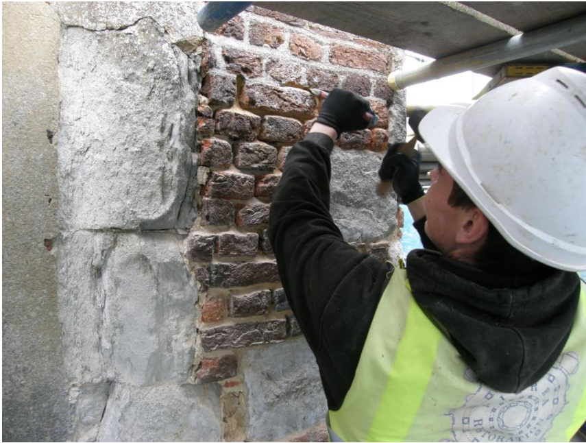
Notice the depth of the cut and the poor state of the stonework
