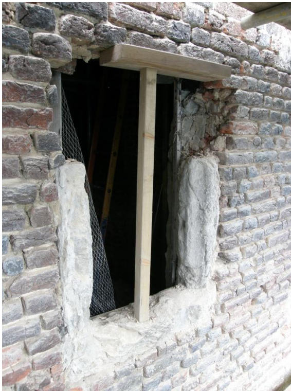
Notice the depth of the cut and the poor state of the stonework
