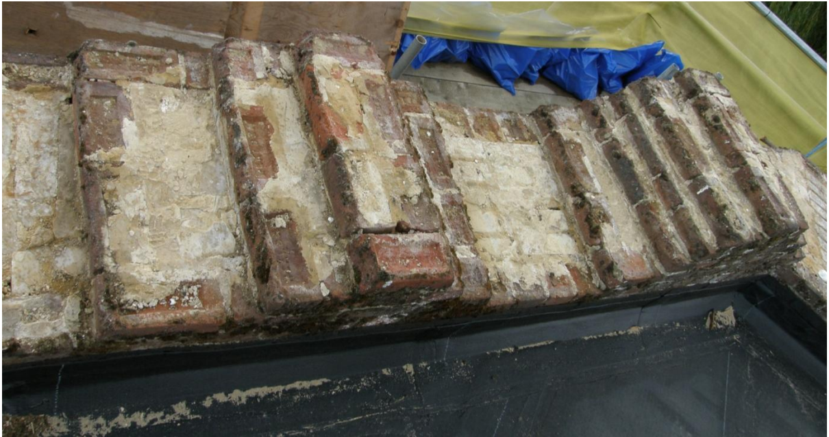
1: The Balustrade with the concrete removed
