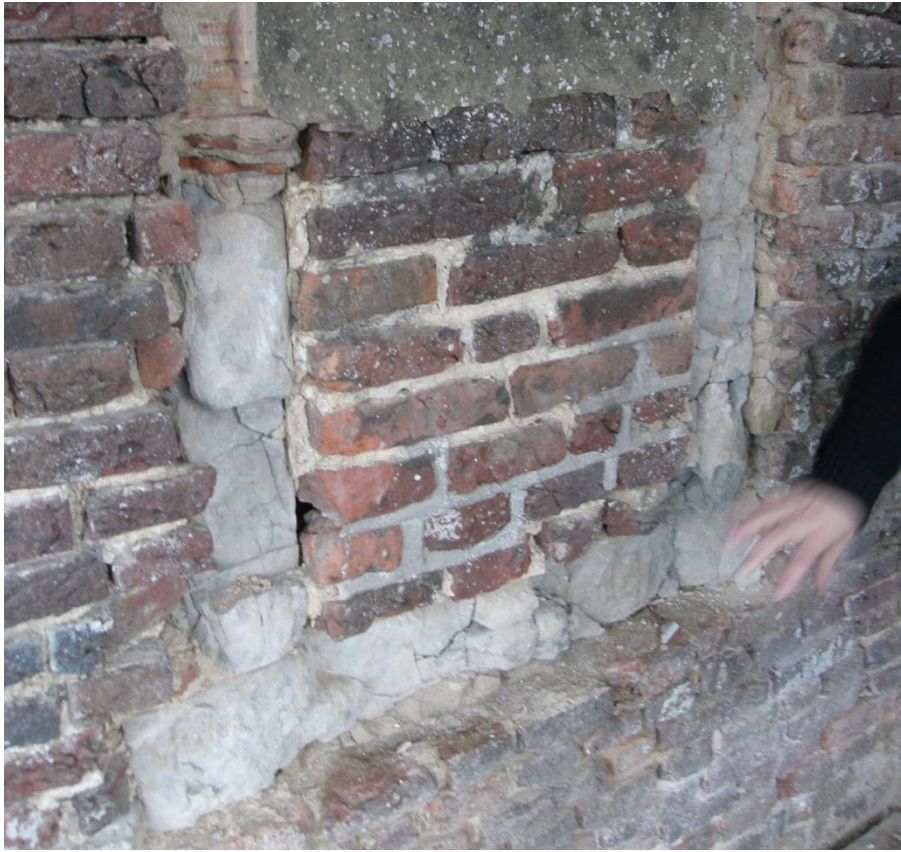
5: Mullions and cil, once single pieces of Kent Rag, reduced to rubble with the effects of a cement coating. Ominous what state parts of the tower had reached even though not previously visible.
