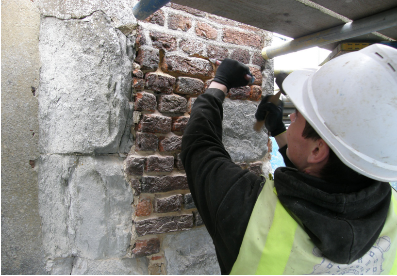
Figure 14: Recent Repair Work To Mortar Joints (2015)
