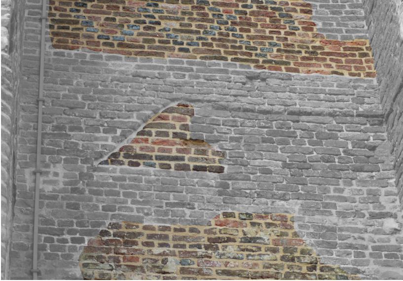
Figure 47: Mortar Repairs To The Tower (2017)
