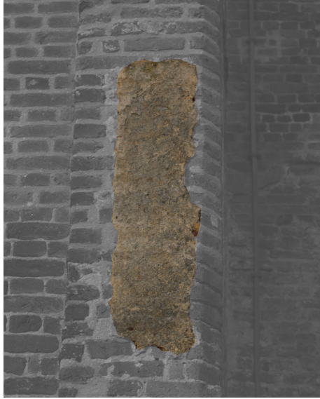
Figure 51: Concrete Repair To Tower (2017)
