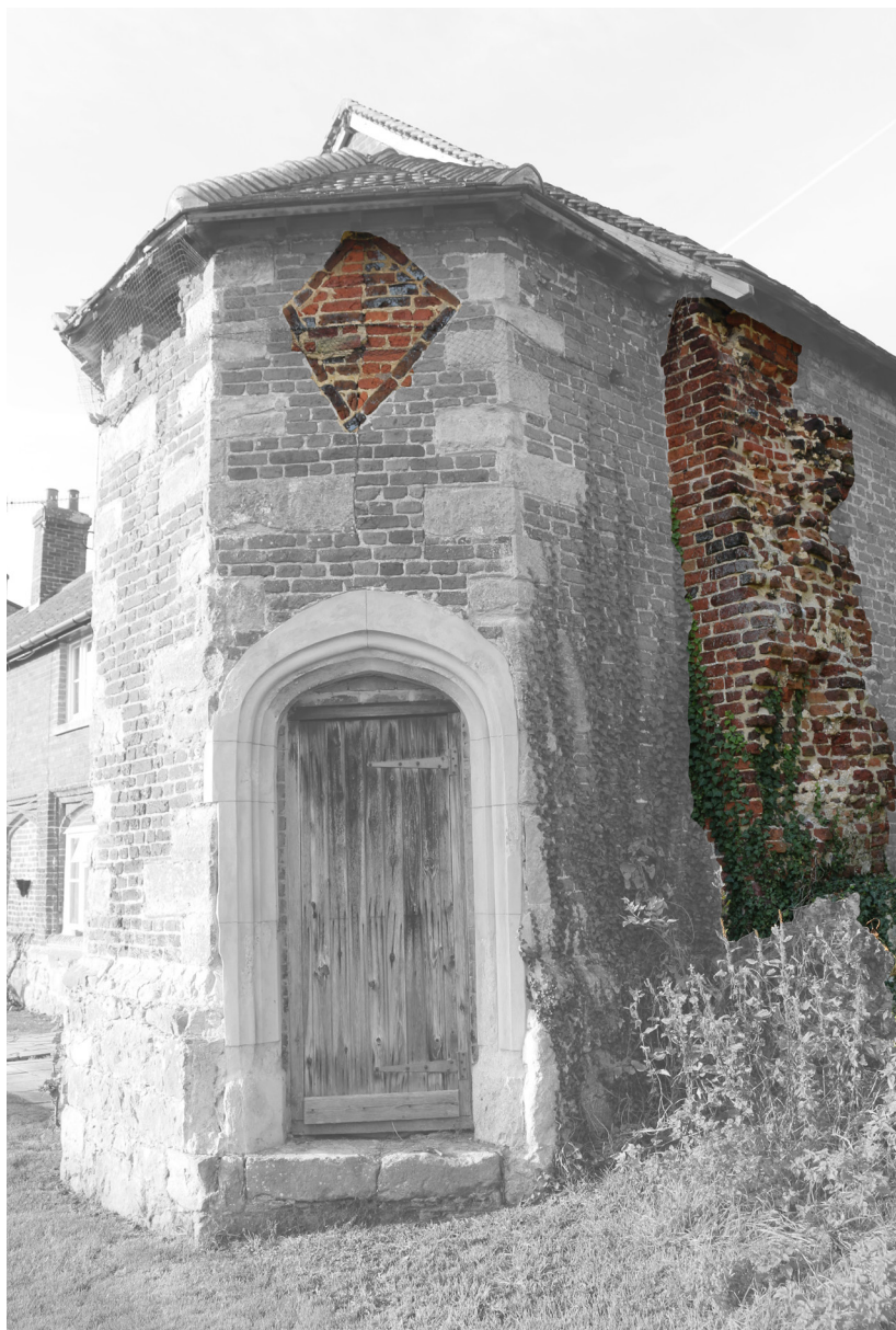
Figure 35: External Patterned Brickwork&Remains Of Brickwork Connections (2017)
