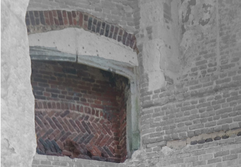
Figure 38: Original Fireplace and Structural Arch (2017)
