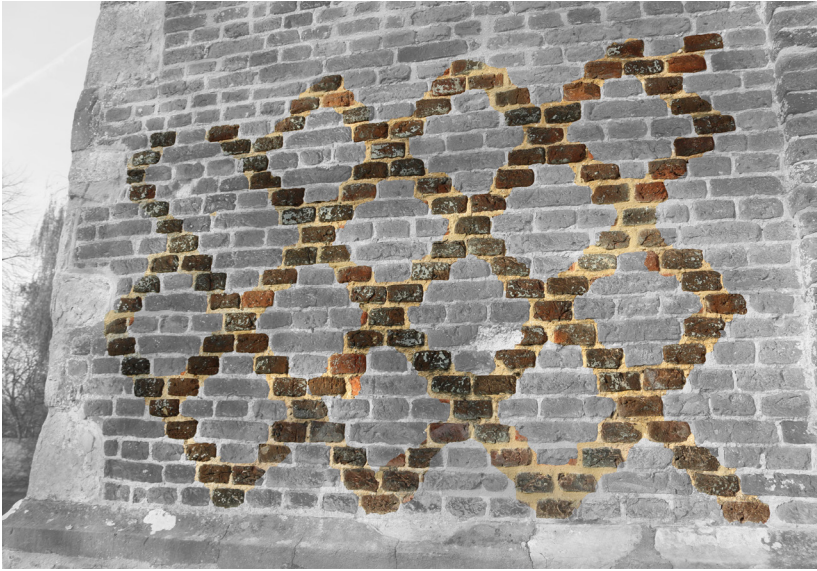
Figure 45: Decorative Burnt Brickwork Pattern (2017)
