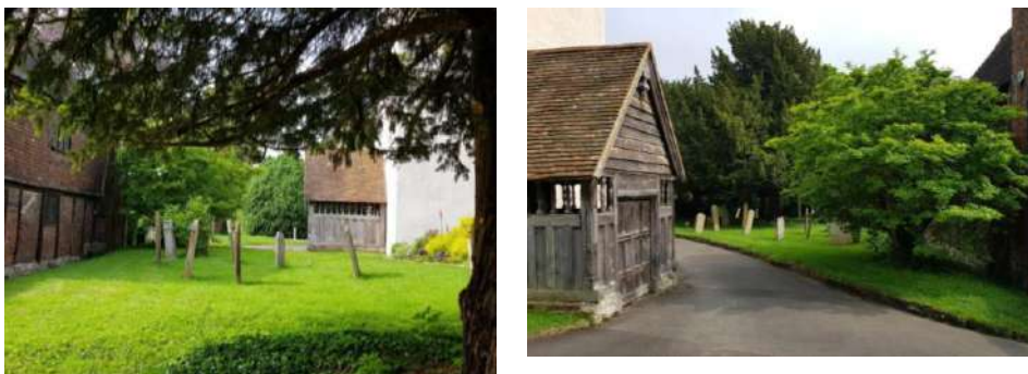
Figure 5: Views looking north with the Church on the right and The Chantry on the left, looking South with the Church on the left and The Chantry on the right. (Photograph, Author 2018)
