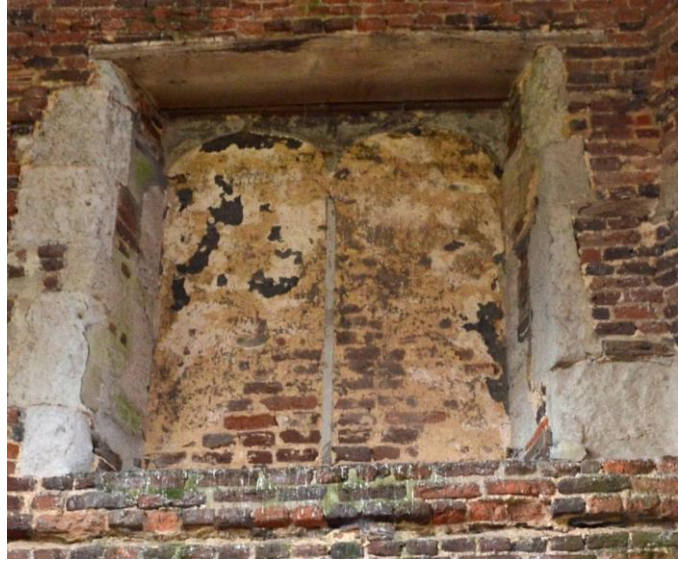
Figure 4: WF/01 on the first floor with brick infill
