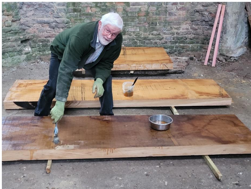
Figure 9: Applying the preservative mixture
