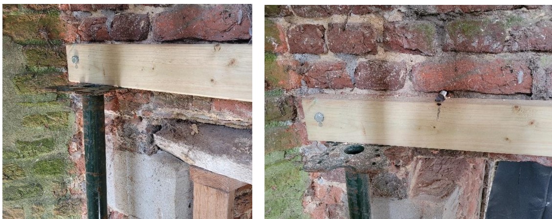
Figure 11: Support for the needles (visible in the right-hand image)
