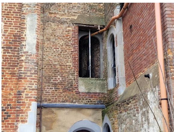
Figure 7: A temporary Acrow prop to support the decayed lintel
