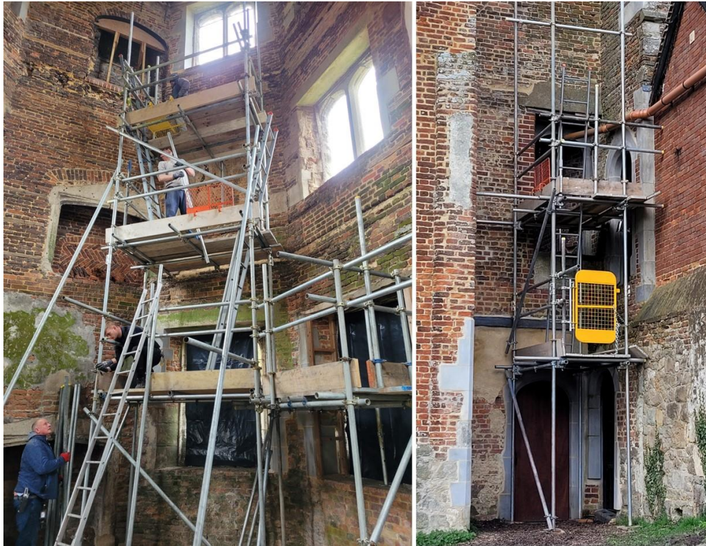
Figure 10: Scaffolding for the lintel replacement - inside and outside
