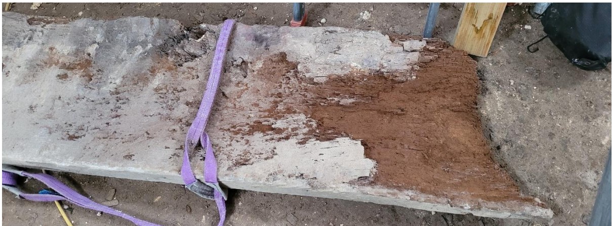
Figure 13: Decay on lintel WG/02
