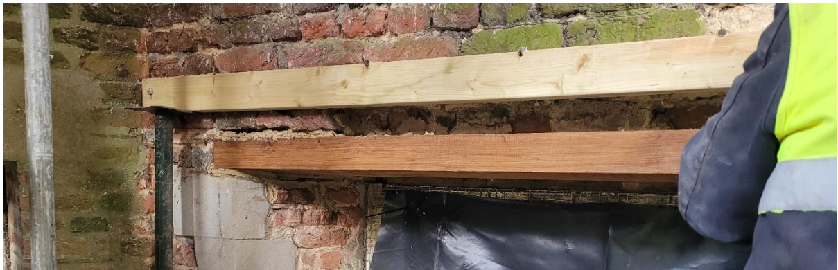
Figure 14: Sliding the new lintel for WG/02 into position
