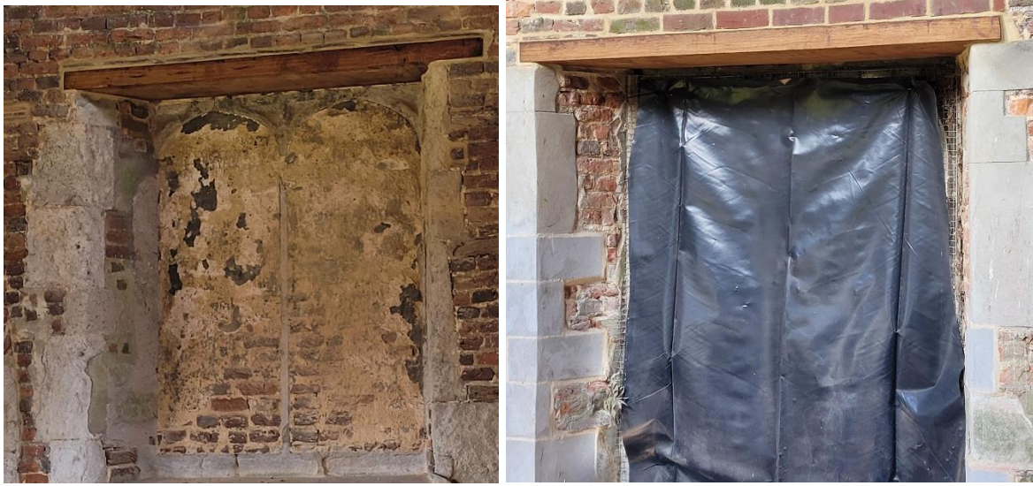
Figure 15: The new lintels WF/01 and WG/02
