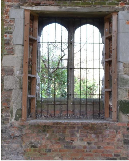
Figure 3: Left: Window WG/02 on the ground floor. Two timber supports.
