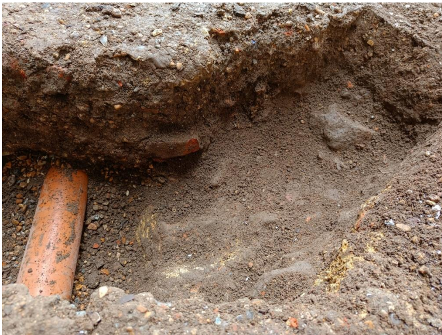
Figure 2: View of the exposed pre-existing drain looking south from the door threshold. This picture shows more clearly that this drain has been cut in to a metallised surface and embedded in a bed of shingle. The smooth surface seen here is to the right (east) of the drain
