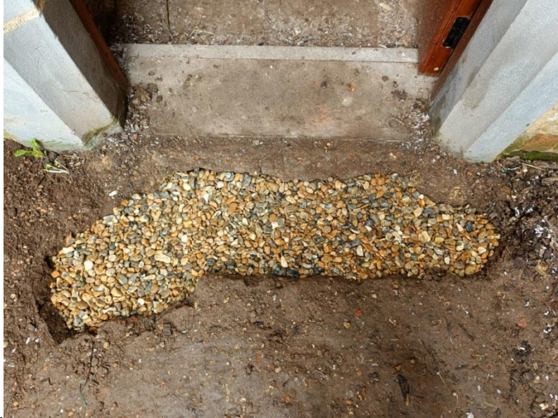
Figure 3: After the trench was refilled, a layer of gravel was placed on top to facilitate drainage
