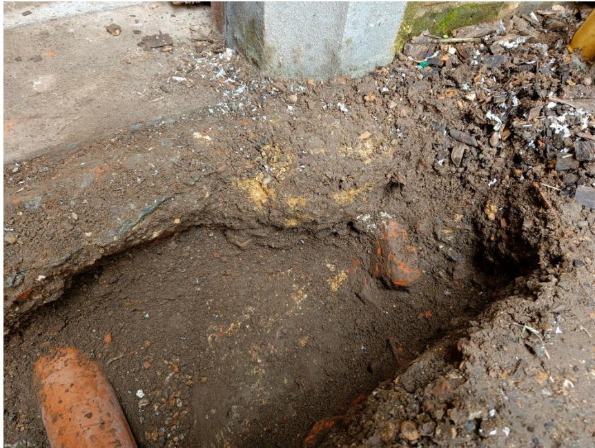
Figure 1: The trench photographed from the south, looking north toward the door threshold. The cement and mortar in the top layer to the south of the threshold had already been removed, presumably when the water-drain seen on the left (beneath centre of door) was originally inserted
