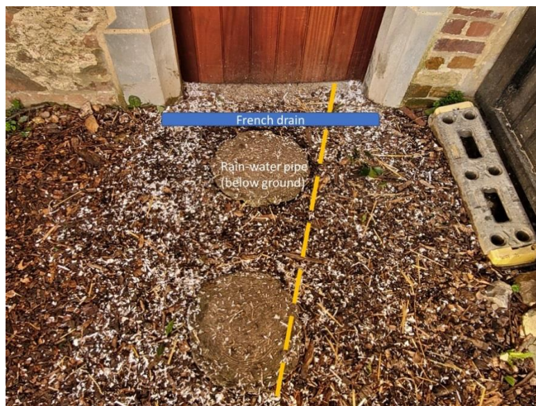
Figure 9: Position of French drain
