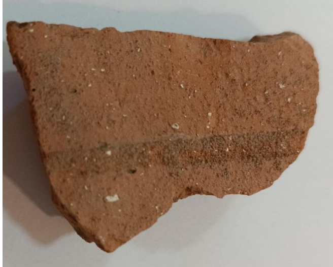
Figure 6: Roof tile showing strike-fault
