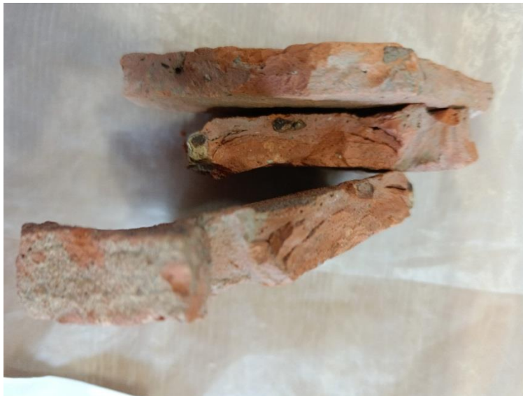
Figure 5: Roof tiles seen edge on. The irregular undulating surface and the crude construction with fabric inclusions are suggestive of medieval manufacture
