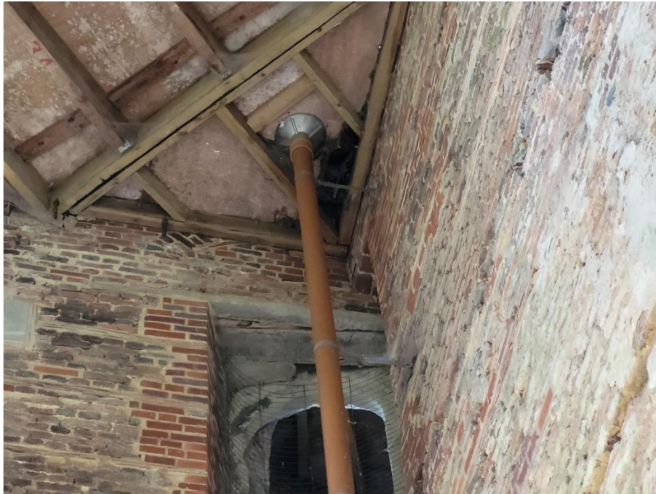
Figure 13: Underside of the roof in the south-east corner showing water damage
