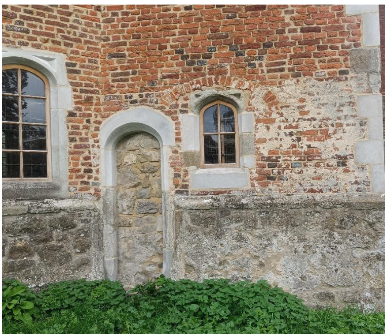
Figure 28: 2025 photograph of external western wall of NW Tower garderobe. To the right (south) of the small window there are the remains of a plaster coat. Could there have been a lean-to building here?
