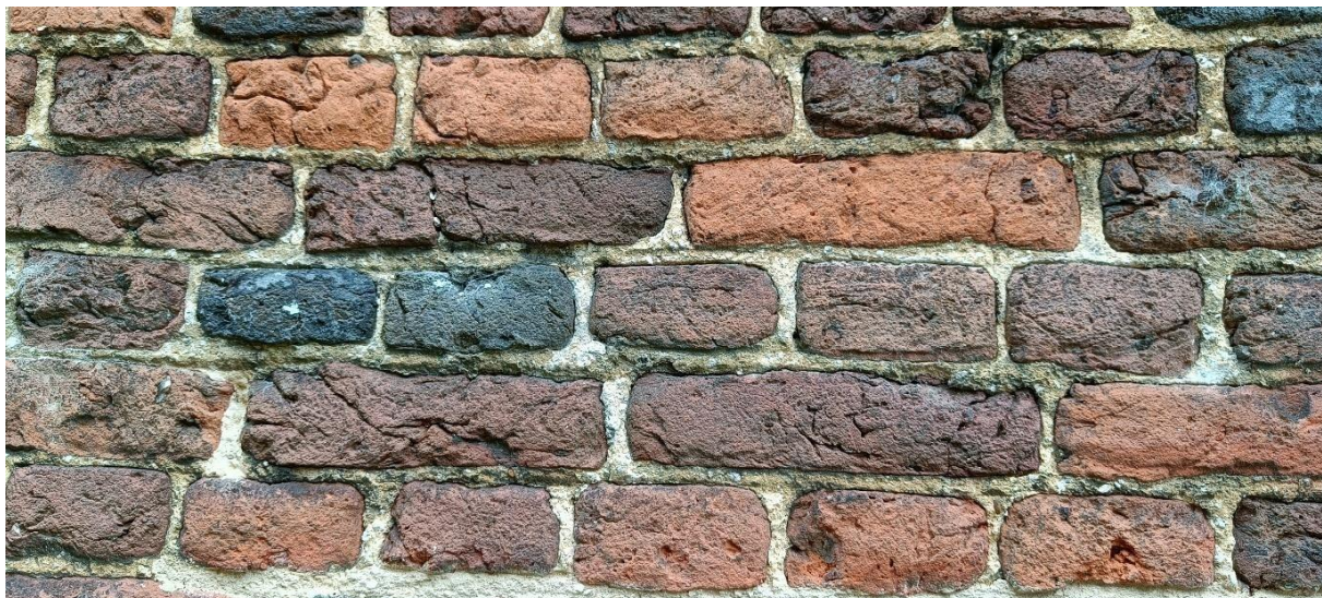
Figure 25: The Tudor bricks on the NW Tower show a variety of colours such as pale orange, orange/red, purple and black/vitrified.
