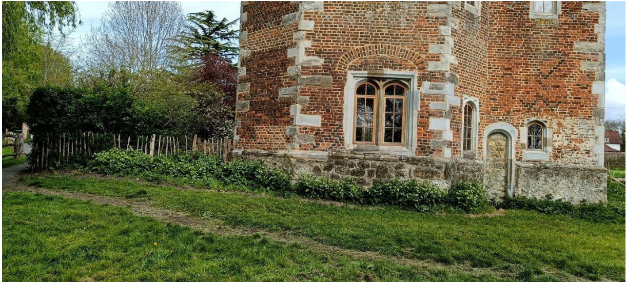
Figure 11: A view of the site of trench 4, taken after it was refilled. The trench ran from the fence post on the left, across in front of the garden of Cottage 1, then close to the western base of the NW Tower, to end in front of the blocked door of the Garderobe
