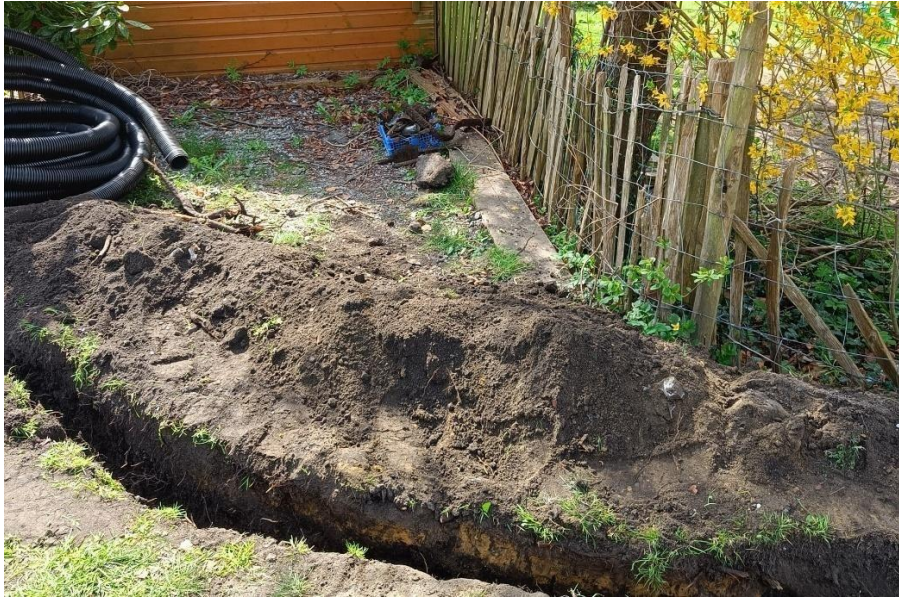
Figure 14: Trench 2 contained a deposit of light-coloured sand, seen just below the surface in the bottom centre of the picture. The protective coil to be used for the electric cable can be seen on the left.
