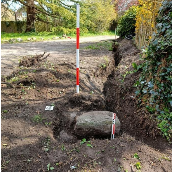
Figure 16: The ragstone at junction of trenches 2 and 3
